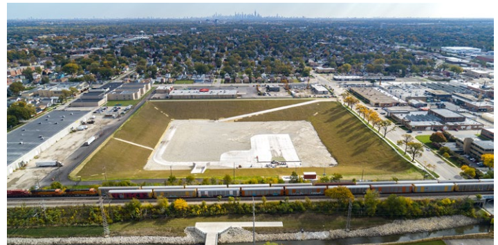
The Addison Creek Reservoir provides 195 million gallons of storage capacity and connects with the Addison Creek Channel (at bottom). Photo taken October 2022.
