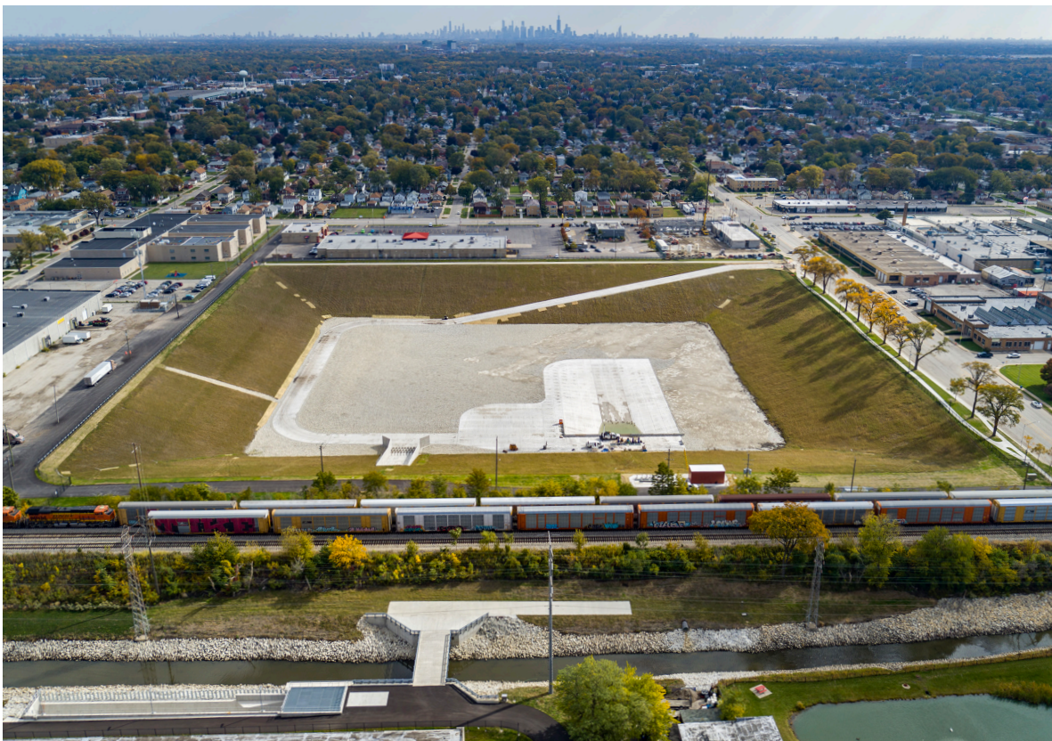
LEFT: The MWRD completed construction of the Addison Creek Reservoir and formally opened it at a ribbon cutting in August 2023. The 600-acre-foot reservoir will hold close to 200 million gallons of stormwater and, along with the Addison Creek Channel Improvement project, will help alleviate public health and safety concerns by reducing overbank flooding to approximately 2,200 structures along the creek for businesses and residents in Northlake, Stone Park, Melrose Park, Bellwood, Westchester and Broadview.
