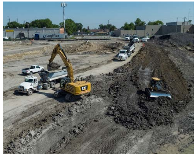
Excavation at the Addison Creek Reservoir in Bellwood, Illinois.
