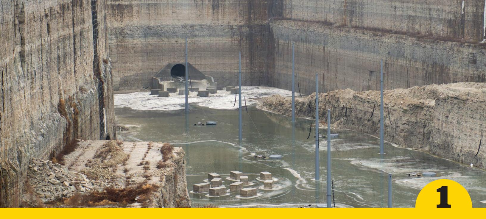
Water rushes into McCook Reservoir Stage I. Baffle blocks built at the tunnel openings prevent the force of the water coming out of the tunnel from eroding the reservoir floor.
