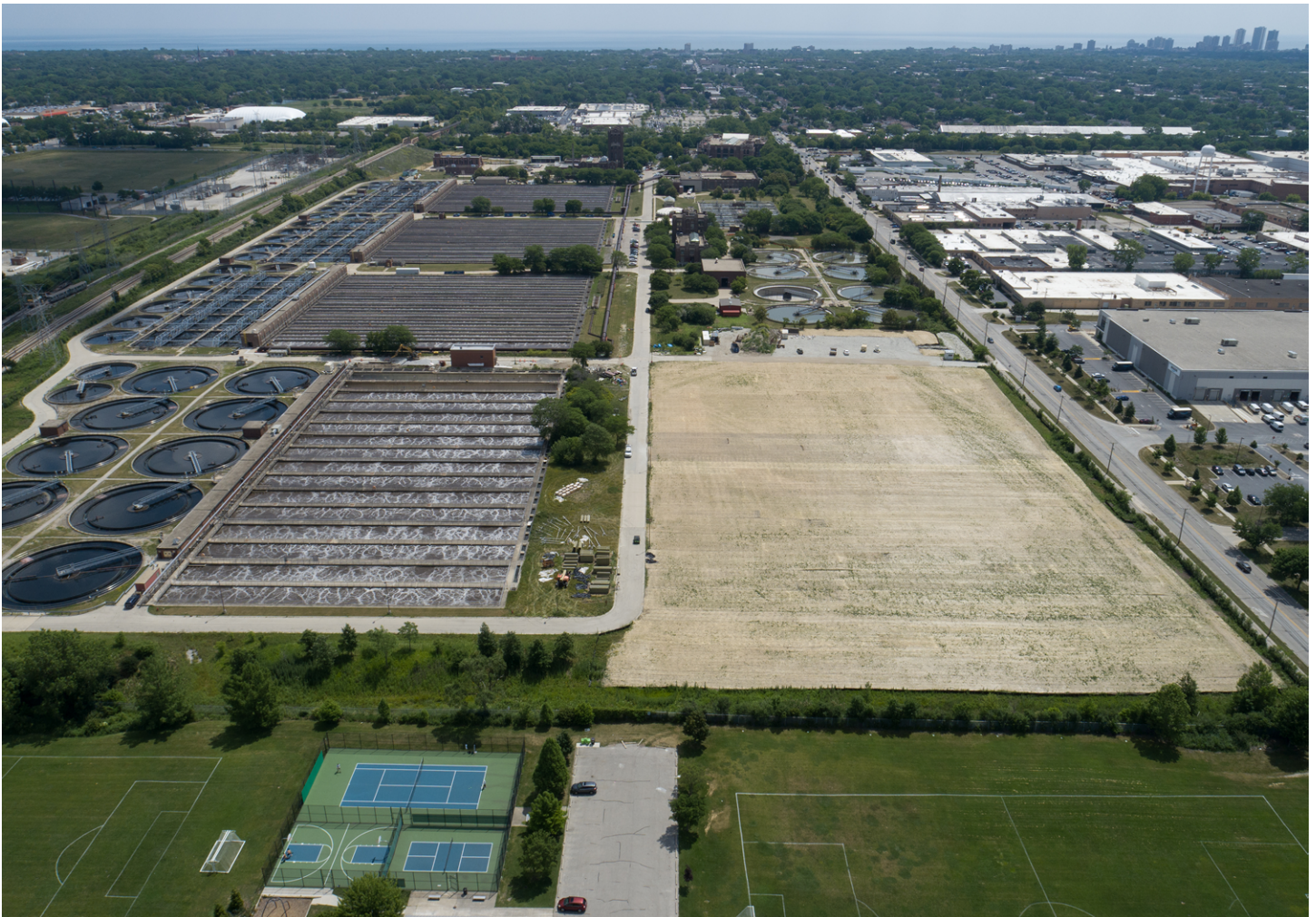
The MWRD is clearing ground on the southwest side of its O'Brien Water Reclamation Plant to make way for new essential infrastructure that will replace aging facilities and help improve the water reclamation process by removing more phosphorus from wastewater using a biological process that meets new permits and better protects water quality downstream of the North Shore Channel.
