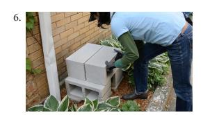
"Getting the barrel up and off the ground will increase the water pressure coming out and will make it easier to fit buckets and watering cans under the spigot. A full 55-gallon barrel will weigh about 500 pounds, so the platform needs to be strong and stable. We're using a few cinder blocks which are very affordable."
