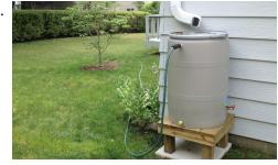
"Rain barrels can fill quickly during a normal rain storm. So we need to be prepared to direct that overflow water to absorbant ground away from your home and your neighbors. Run a hose from the top of the barrel into your yard or garden."
