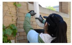
"Connect the diverter to the cut downspout. Be sure the diverter is properly and firmly attached with sheet screws and the upper section is inserted into the lower section."
