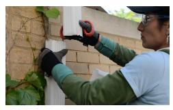
"Double check your measurements before you cut because this is the point of no return! Put on your safety goggles and gloves and cut the downspout with a hacksaw or tin snips."
