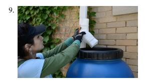
"Position the flexible diverter elbow on top of the barrel aimed at the screened opening and next to the downspout to determine where to cut."
