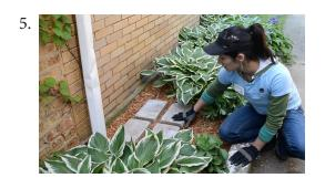
"We've prepped this area with mulch in order to absorb any water that comes off of the rain barrel. And we've evenly spaced these pavers so that water can infiltrate through and reach the mulch. When we cut the downspout, there's going to be a hole and we're going to need to cover the hole so no debris clogs the sewer."
