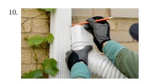
"The remaining downspout will need to be inserted about two inches into the elbow, so you can make a reference line next to the top of the elbow..."
