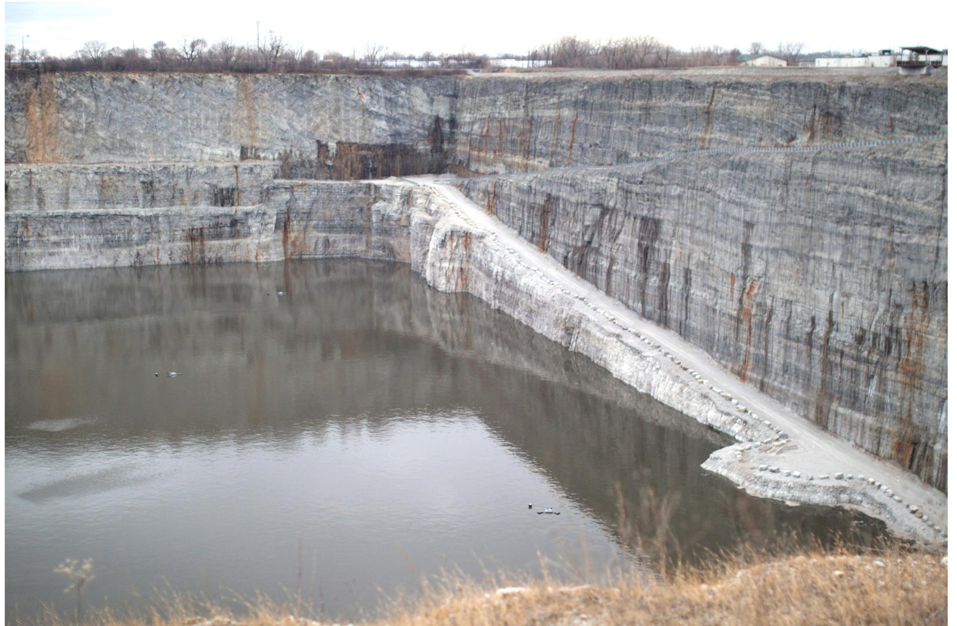
*Beginning on November 26, 2015, the Thornton Composite Reservoir began to fill for the first time. It reached 17 feet and contained 400 million gallons of combined sewer overflow prior to being transported by tunnel for treatment at the Calumet Water Reclamation Plant.*
