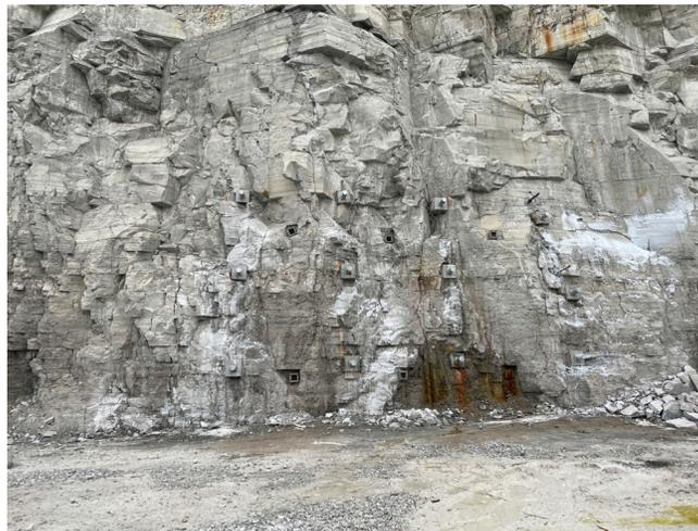
*Rock anchors and drain holes provide additional stability to key blocks of the rock wall at the Thornton Rock Dam .*
