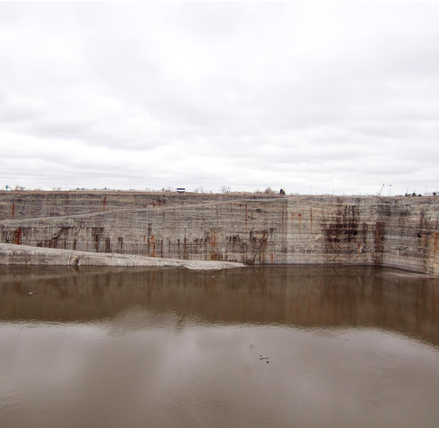
*The Thornton Composite Reservoir prevents combined sewage and stormwater from entering and overwhelming Calumet area waterways. It contains the water before it can be conveyed by tunnel for treatment at the MWRD's Calumet Water Reclamation Plant. Since 2015, the reservoir has captured about 59.1 billion gallons from flooding local sewers, polluting waterways and backing up into local basements.*
