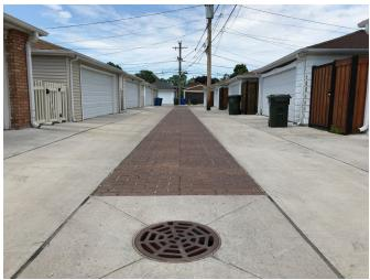
A green alley in Harwood Heights, funded by the MWRD, collects precipitation where it falls by detaining and infiltrating runoff to prevent it from overwhelming sewers and flooding communities. The MWRD will contribute additional funds to expand green alleys in Calumet City, Des Plaines, Lyons and Maywood among other community projects in 2022.
