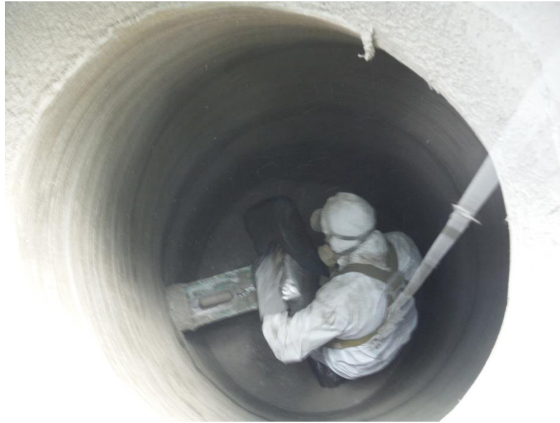
Figure 8.18: Manhole Rehabilitation by Cementitious Lining
