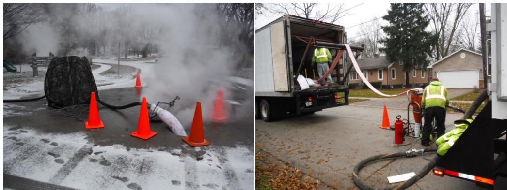
Figure 8.19: Cured-in-Place Pipe (CIPP) Lining
