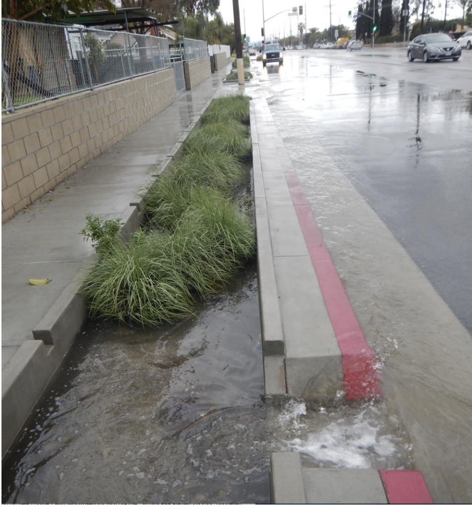
Laurel Canyon Blvd, Los Angeles Los Angeles Dept. of Water & Power
