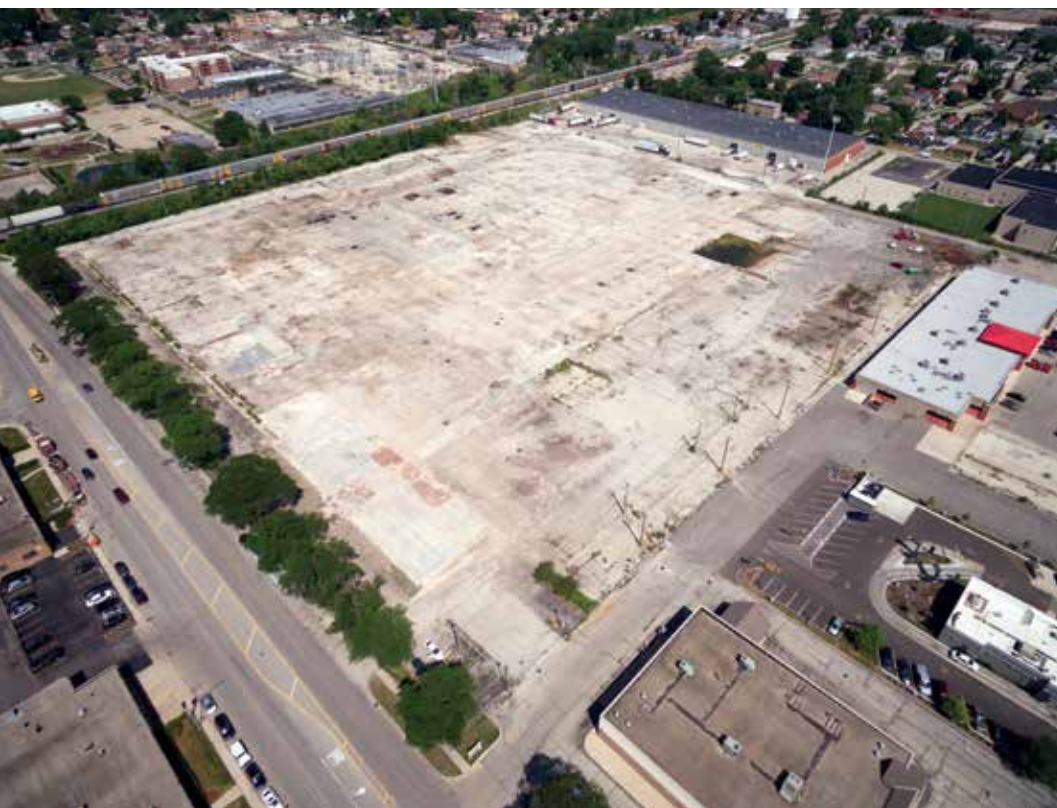
Addison Creek Reservoir. 11-186-3F
