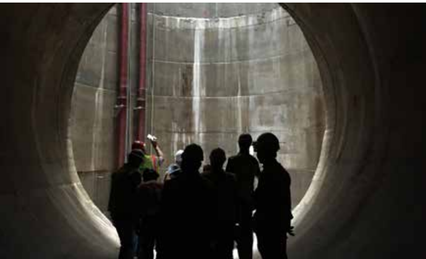
Albany Park Stormwater Diversion Tunnel (Contract: 14-066-3F). Rising water flows through the grated areas into the tunnel, coming out further downstream. This keeps the water levels from rising and causing a flood.
