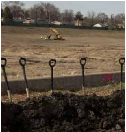
Melvina Ditch Reservoir Improvements. 14-263-3F
