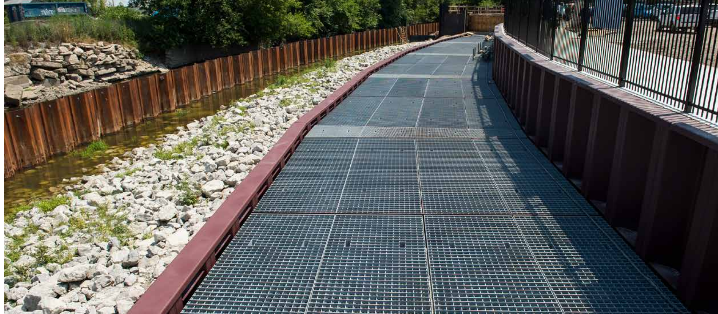
Albany Park Stormwater Diversion Tunnel (Contract: 14-066-3F). Rising water flows through the grated areas into the tunnel, coming out further downstream. This keeps the water levels from rising and causing a flood.
