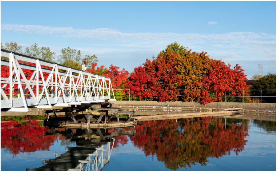
Primary Tanks at the Calumet Water Reclamation Plant.
