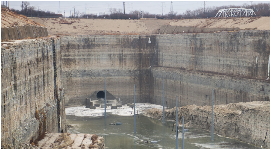
First fill at McCook Reservoir Stage 1.
