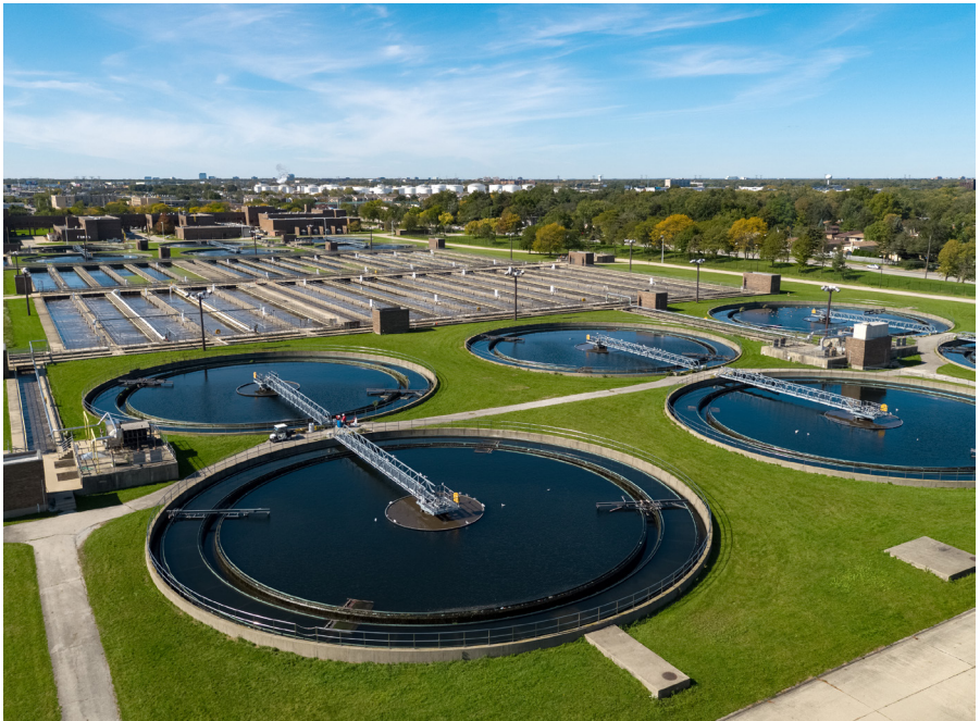
James C. Kirie Water Reclamation Plant in Des Plaines, IL.
