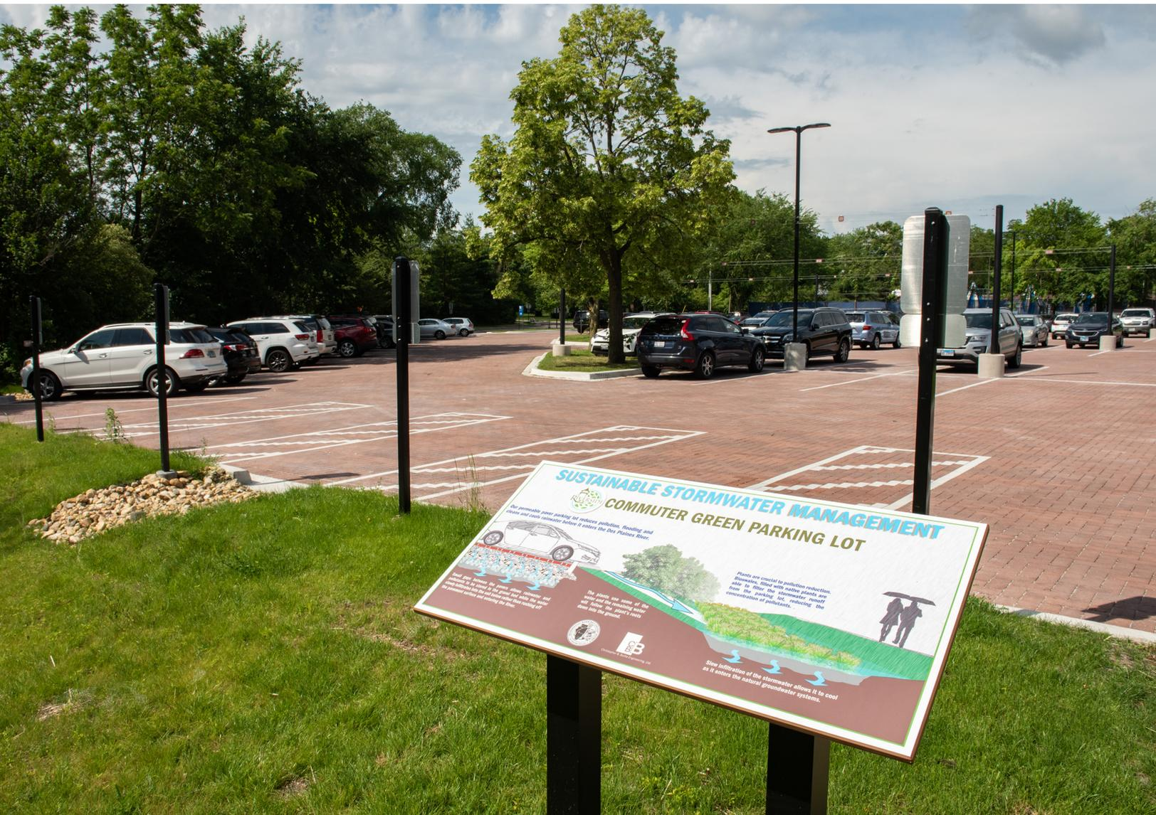
The District partnered with the Village of Riverside to construct a new commuter parking lot and bioretention area that will provide parking for Metra commuters and more than 237,000 gallons of stormwater storage per rain event. The permeable parking lot and rain garden will reduce the current load to the combined sewer system and help alleviate flooding within the project area.
