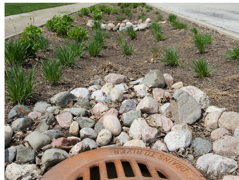
The MWRD promotes green infrastructure projects that use natural landscaping to manage water.
