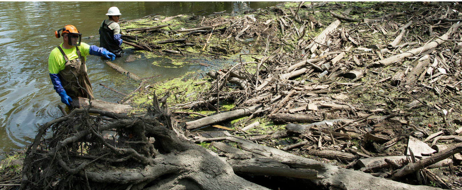
A crew removes a logjam in the North Branch of the Chicago River as part of the MWRD's Small Stream Maintenance Program.
